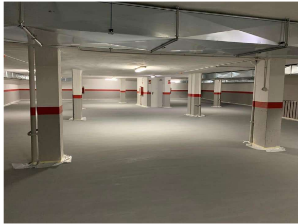
2- Resiepoxy layers application
